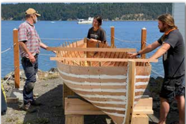
An instructor gives guidance to students Courtney and Mo as they fasten red cedar planks to oak frames on a 14' Davis double ender using rivets and roves.
